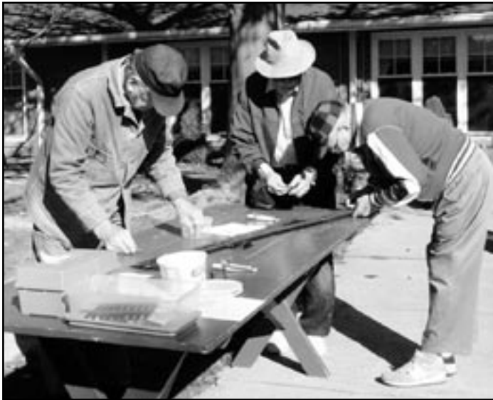
Ken Noll, Luke Bomberger and Frank Wilson work on track.
