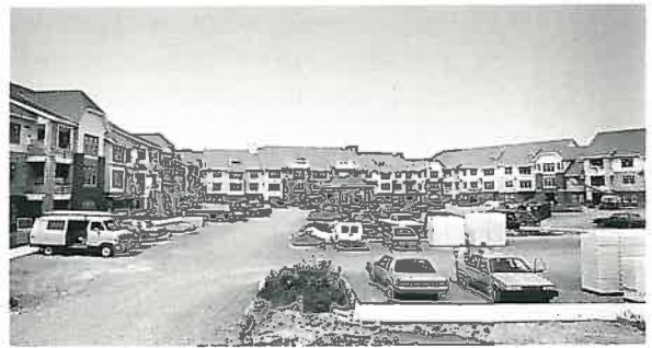
Harvest View under construction.
